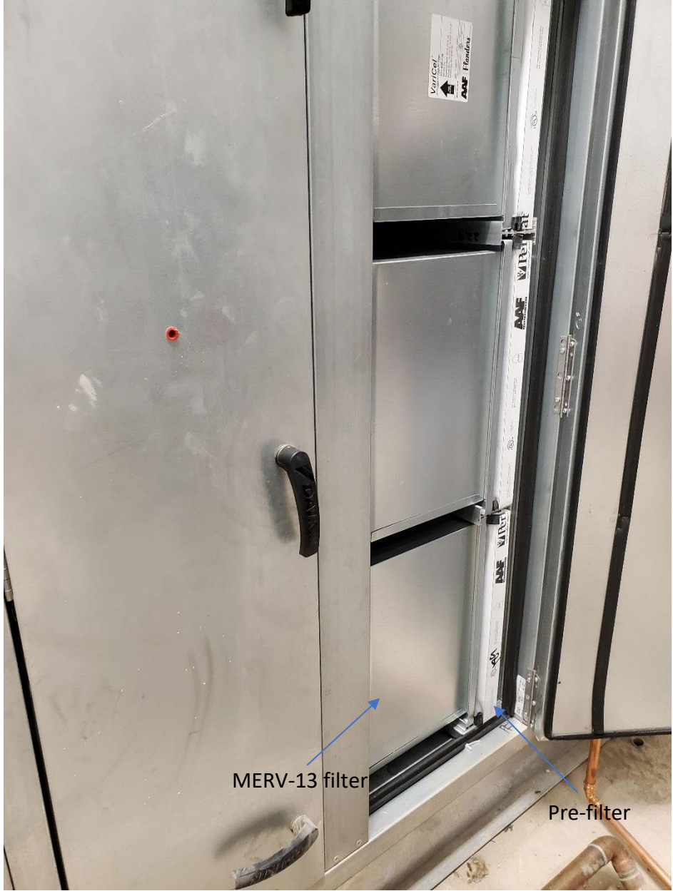
MERV 8 pre-filters with MERV 13 box filter in air handler unit
