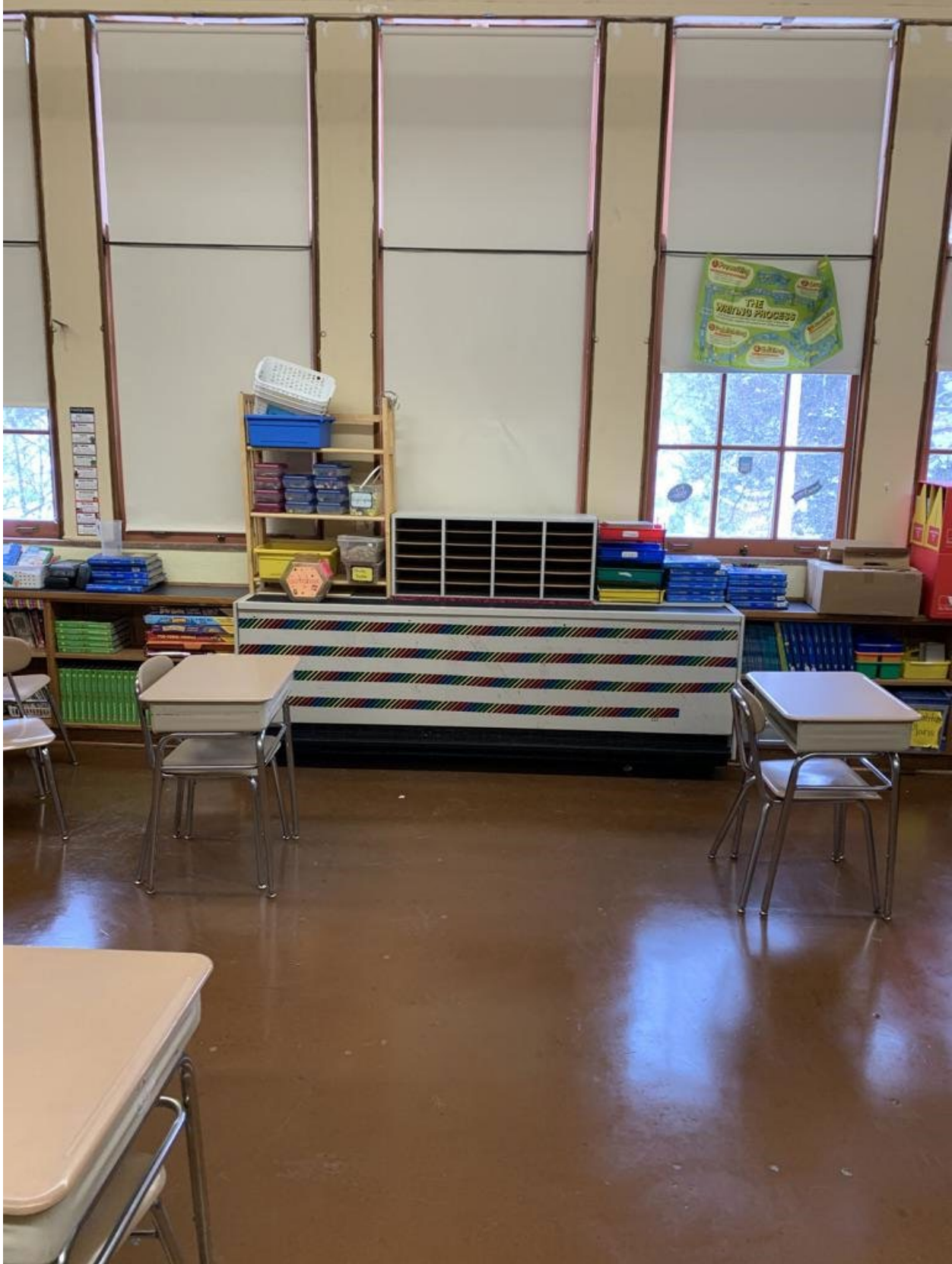
Operable windows and univents – prevent blocking of the vent with stored materials
