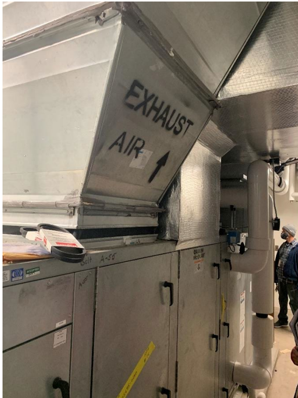
Inside the mixing box of air handler unit serving the new wing. As noted in the report, the unit currently utilizes MERV 8 filters until incoming MERV 13 filter are delivered. To bypass need for filtration, systems are operating to maximum outside air (dampers open) and minimize return air (dampers closed).
