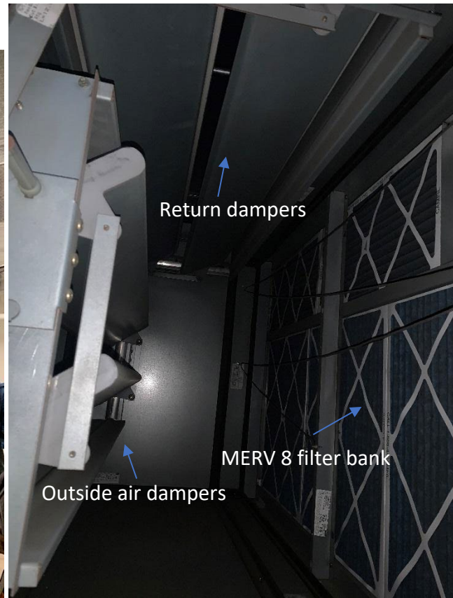
Inside the mixing box of air handler unit serving the new wing. As noted in the report, the unit currently utilizes MERV 8 filters until incoming MERV 13 filter are delivered. To bypass need for filtration, systems are operating to maximum outside air (dampers open) and minimize return air (dampers closed).
