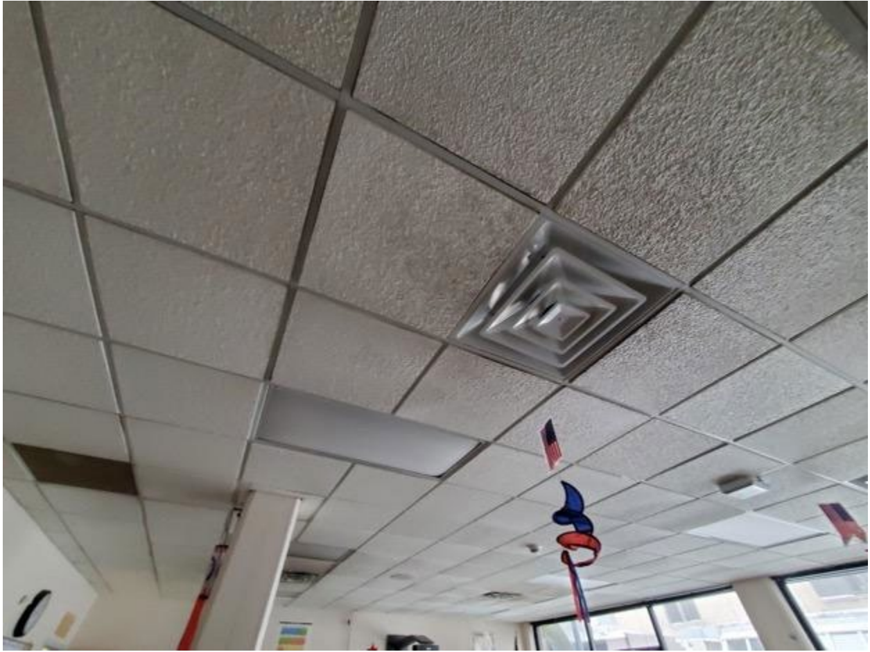
Typical drop ceiling and supply vent in classroom
