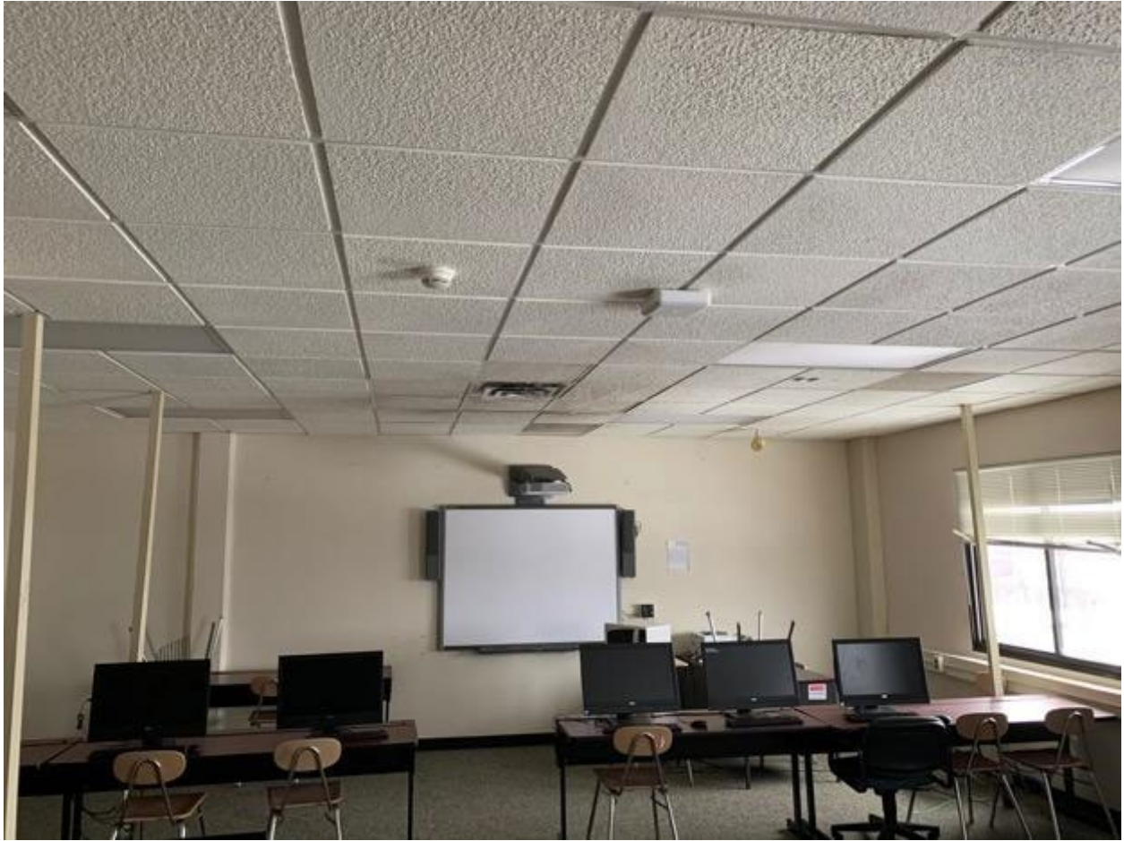
Typical classroom has operable windows and mechanical ventilation
