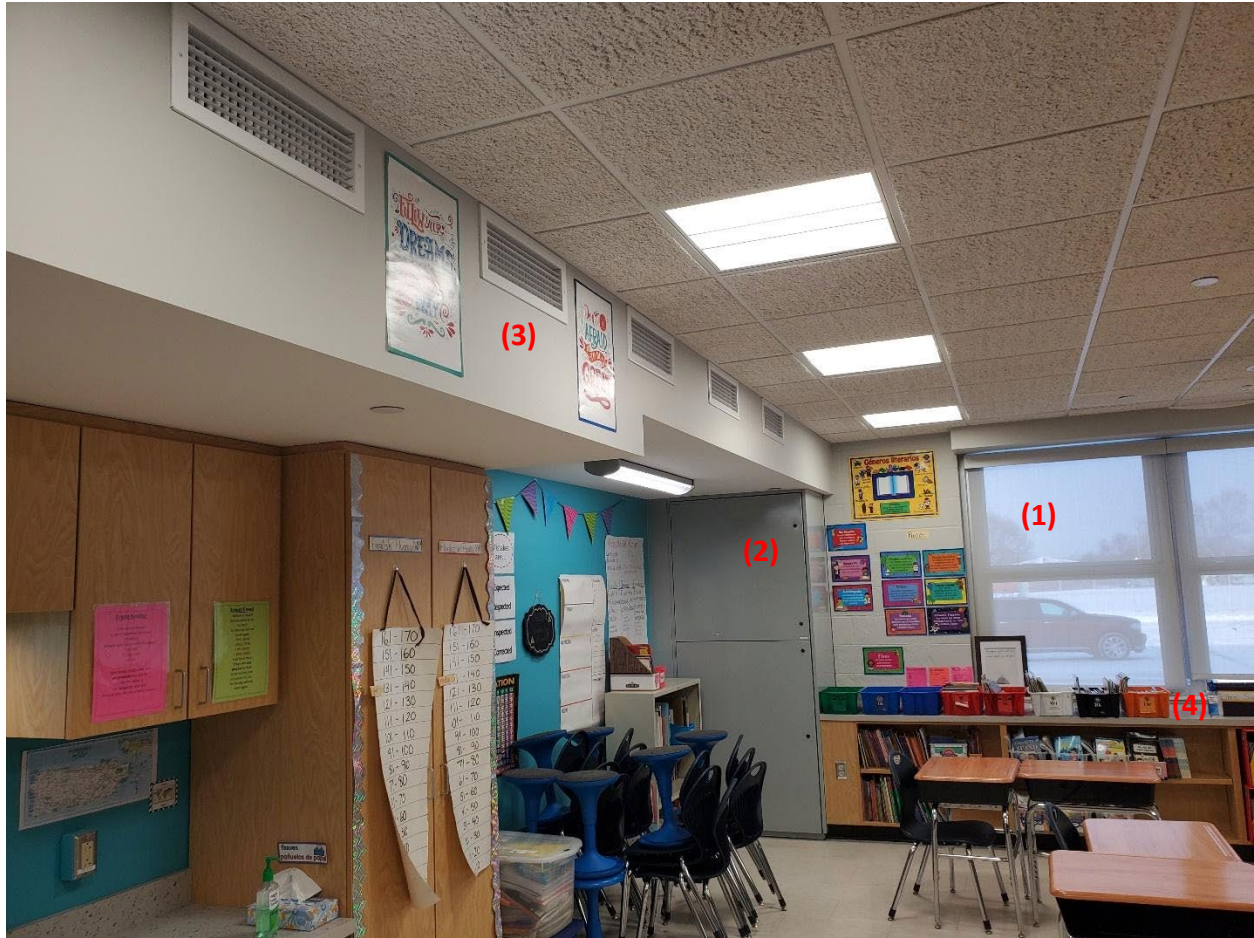
Typical ventilation scheme in classrooms with (1) operable windows, (2) vertical unit ventilator, (3) supply grilles, and (4) return intakes.
