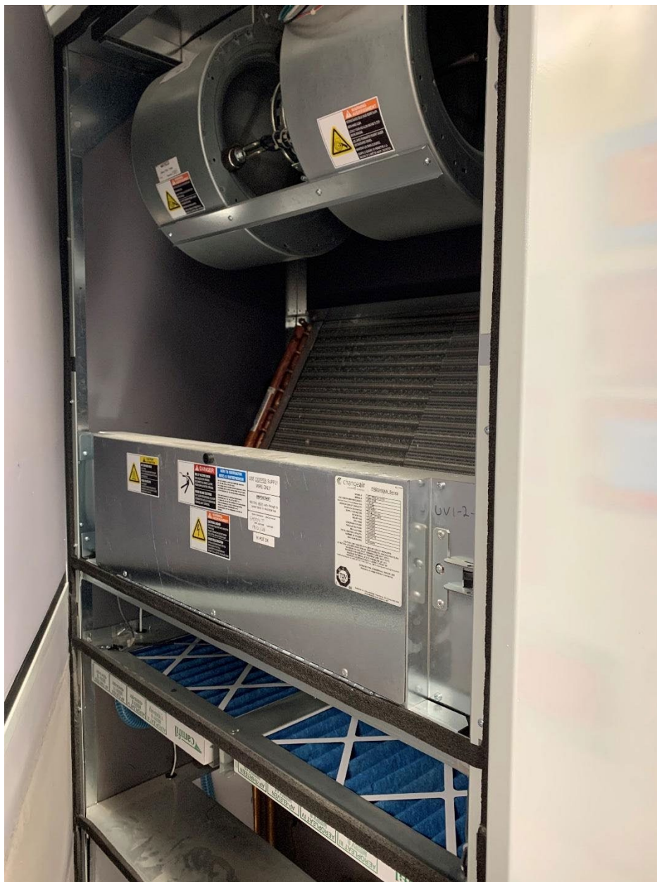
Inside a VUV. Note the MERV 8 (blue) filter.
