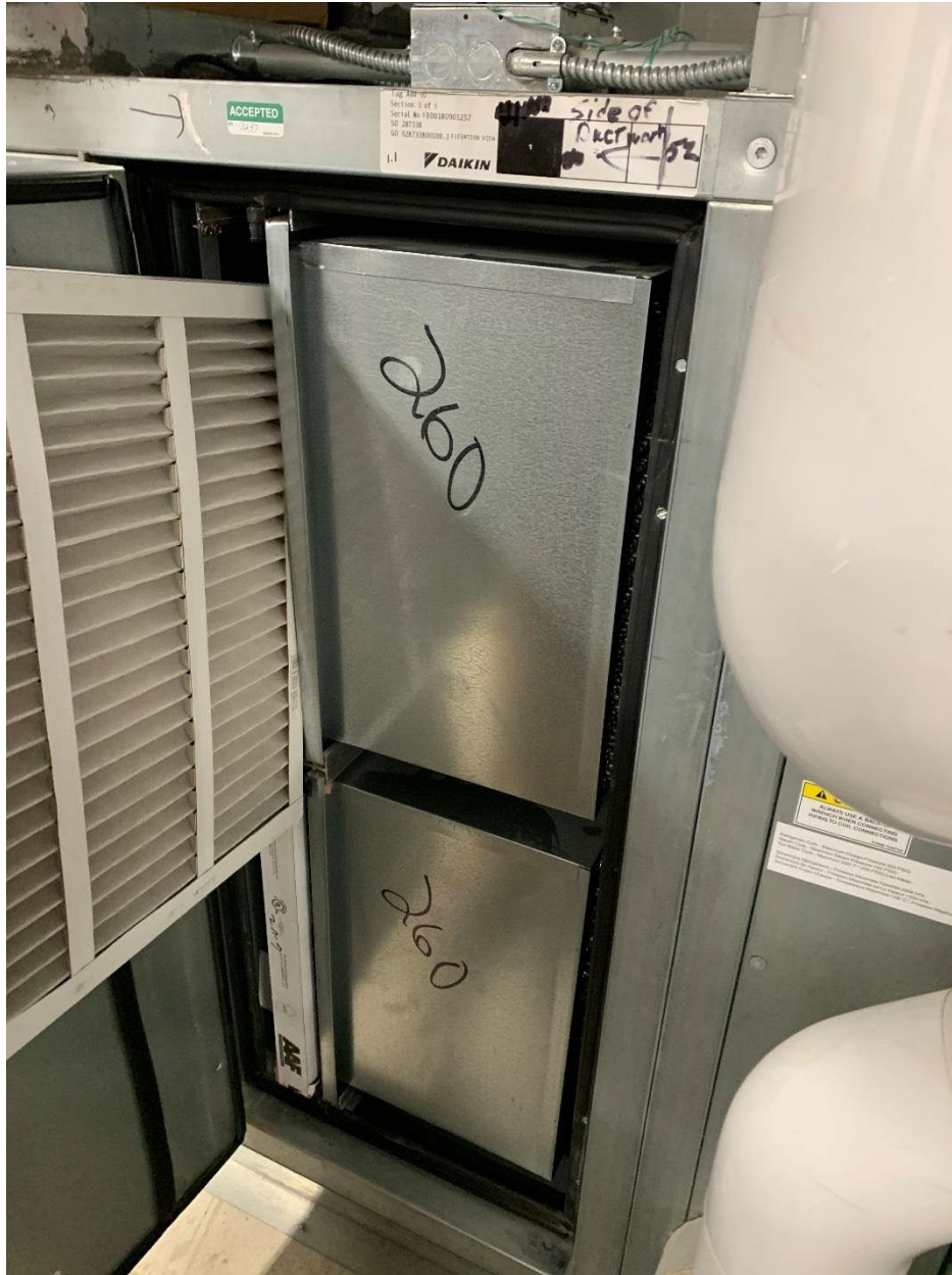
Areas not served by a VUV are served by air handler units. This is the filter bank for an AHU and is typical of the units in the building. They include MERV 8 pre-filters in front of MERV 13 or higher box filters.
