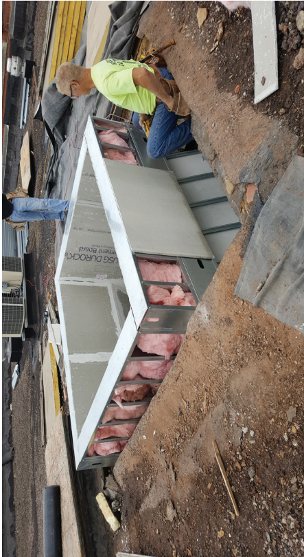
Jefferson – installing new skylight.
