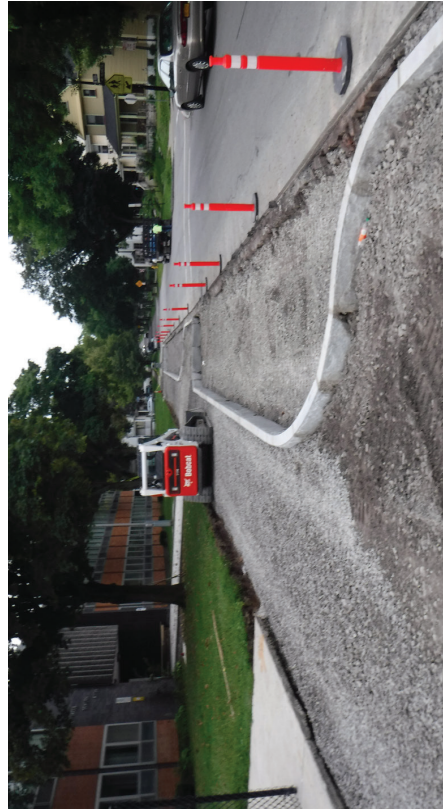
#35 School - constructing bus pull off & new sidewalk.
