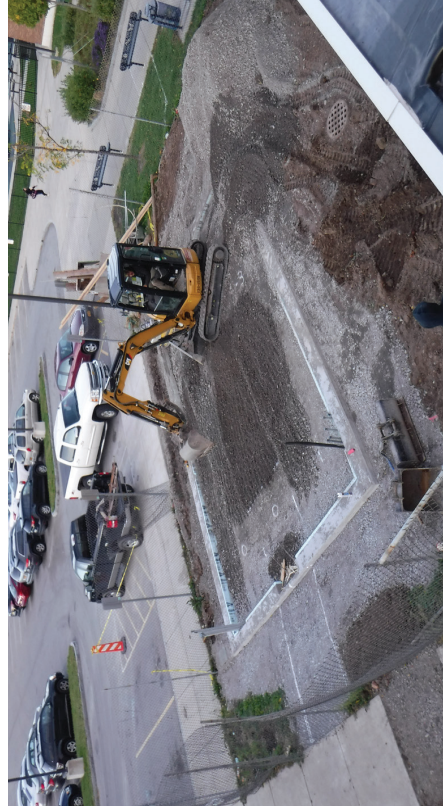
#17 School – constructing foundation for greenhouse.
